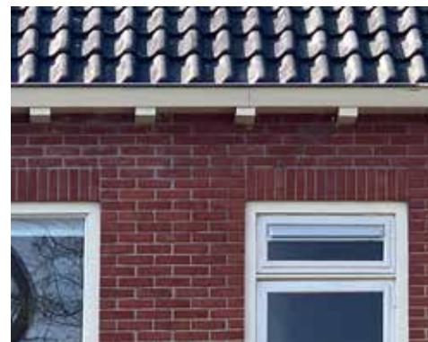
houten bakgoot op houten klossen
